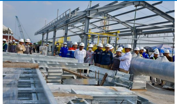
Gambar 5. Proyek Pipa Transmisi Gas Bumi Cisem
